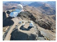
Figure 1: July, 2021 drone photo of the Rubin Observatory summit facility (provided by Dome Surveyor, Oscar Rivera) showing advancement to near 100% on the dome cladding completion as well as closure of the louvers, rear door, and shutters. Sublocation: Cerro Pachón, Chile. Credit: Rubin Obs/NSF/AURA
