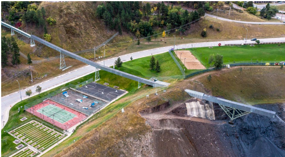
Rock conveyor in operation
