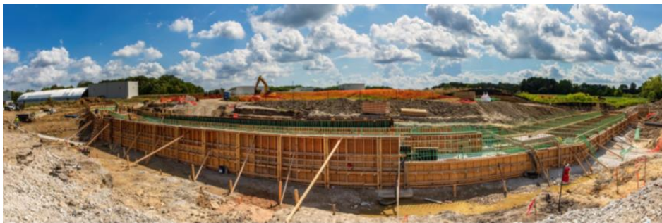
Site preparation for LBNF Beamline facilities completed on schedule in October 2020.
