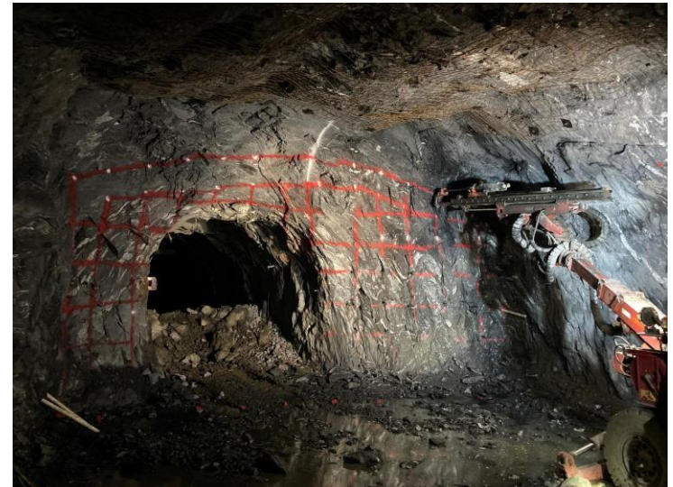
Drilling charge holes
