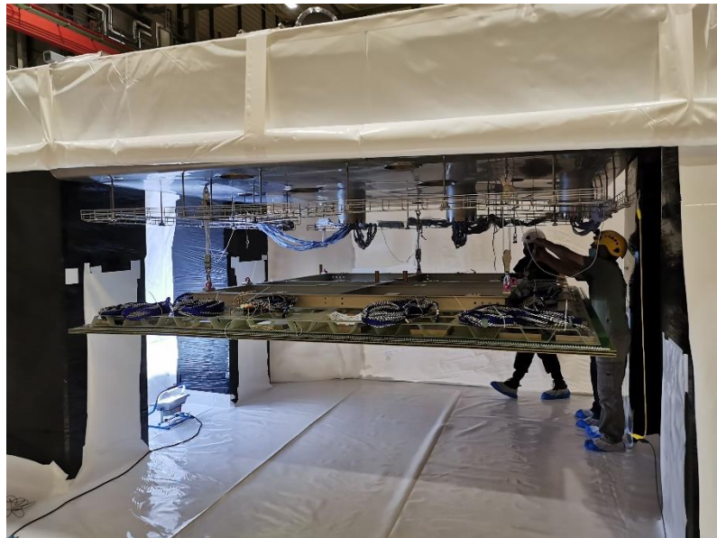
Attachment to the cold box roof
