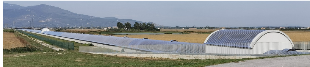
Filter cavity new infrastructure
