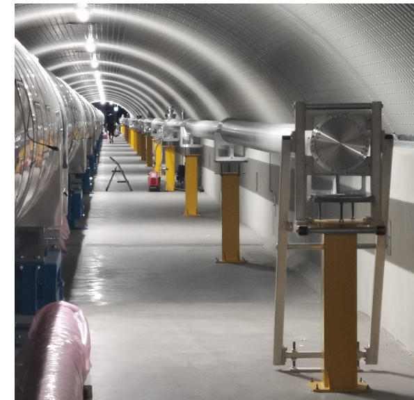
Filter cavity vacuum tube (300 m)
